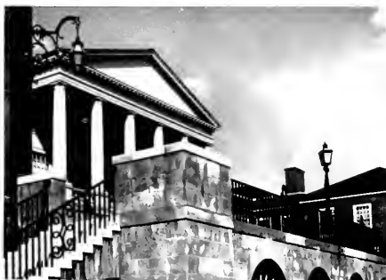
One of our beautiful buildings - Reynolds Hall
